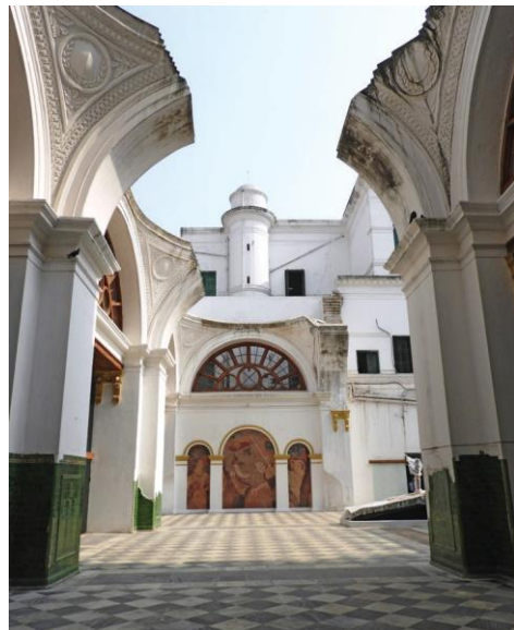
Currency Building, Kolkata, after conservation work by Archaeological Survey of India
